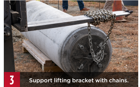
2 Attach lifting bracket to pole base.
