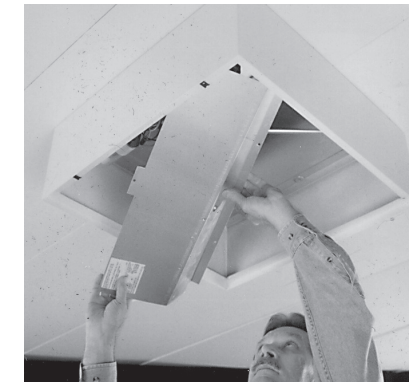
Ballast cover removal
