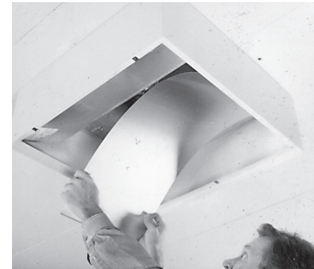
Reflector removal
