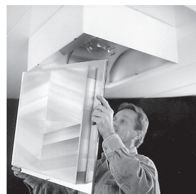
Lens frame assembly removal
